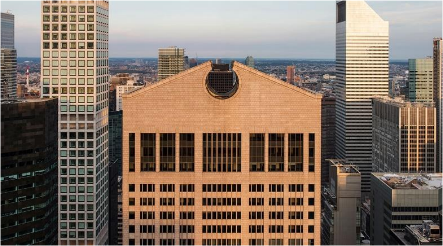
(J) Philip Johnson - AT&T Corporate Headquarters, designed in 1977 and completed in 1984, New York (USA)
